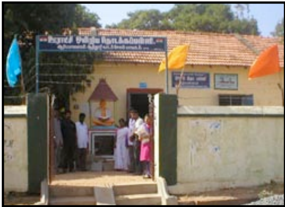
The elementary school entrance.
